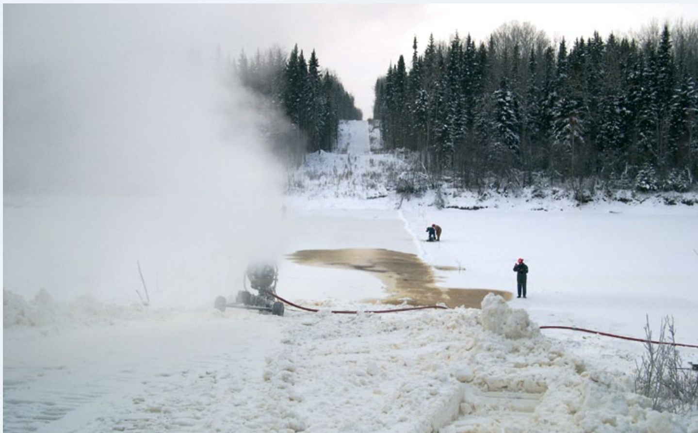
Figure 1. Artificial snow being made at an approach to an ice bridge crossing.
